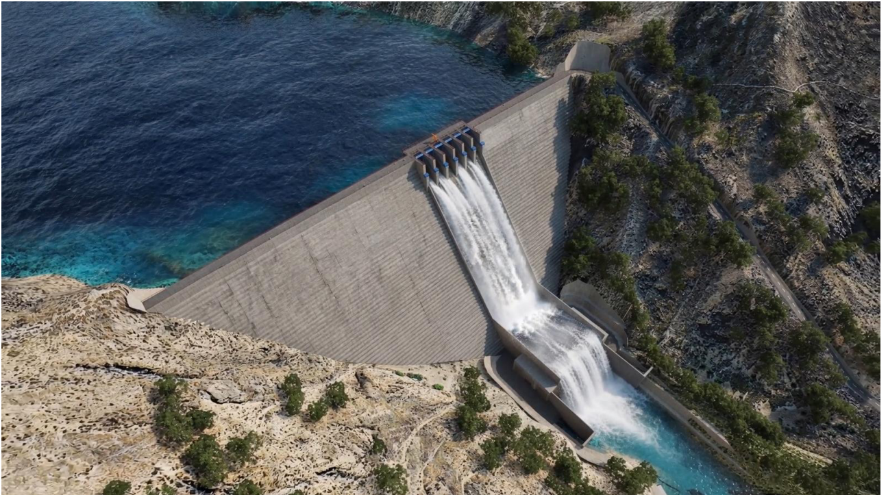
Alabuga Hydroelectric Power Plant
