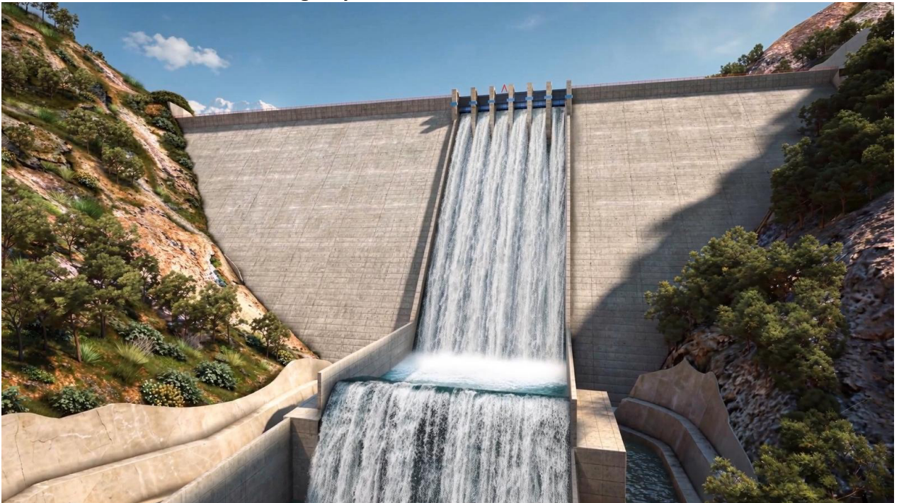
Alabuga Hydroelectric Power Plant
