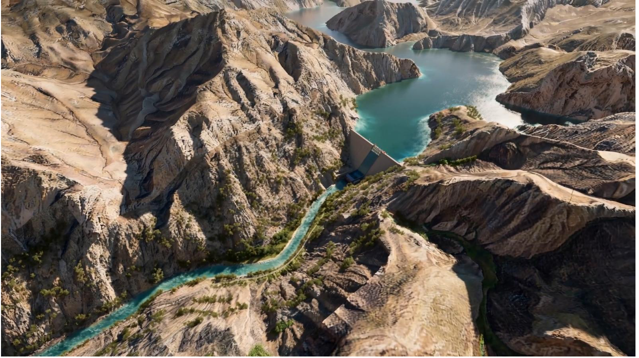
Alabuga Hydroelectric Power Plant
